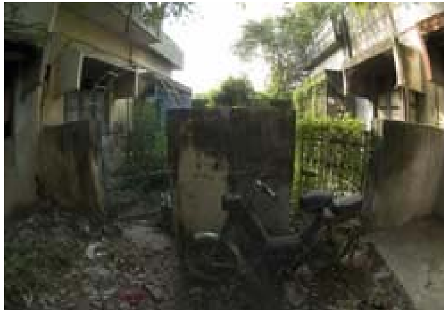
What remains Five years on, the complex is deserted. Photo: Cherian Thomas
