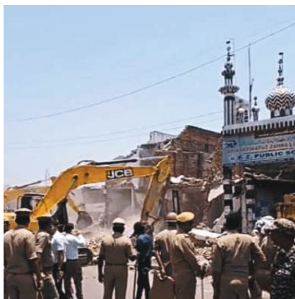
A bulldozer destroys Muslim-owned shops and homes in Lucknow’s Akbar Nagar.
