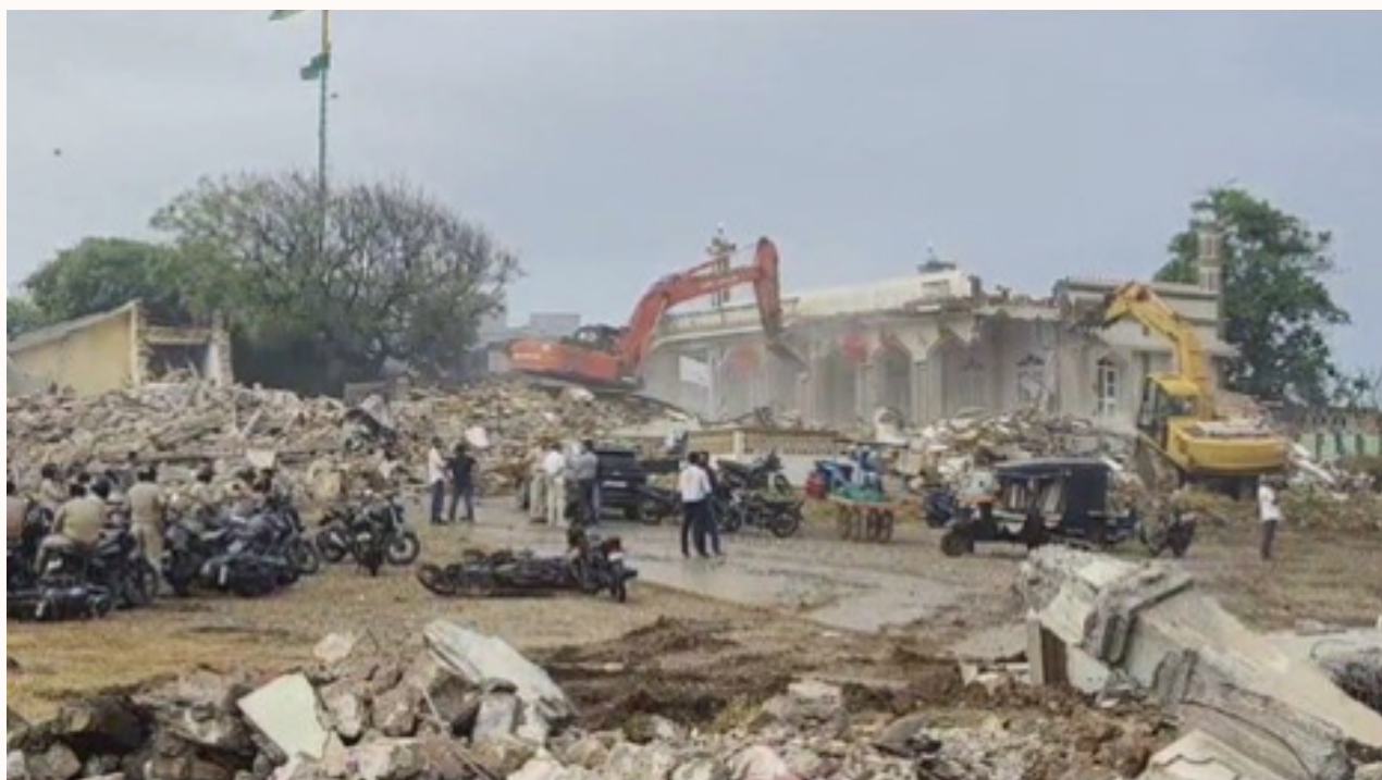
Bulldozers deployed against a historic Muslim shrine in Gujarat’s Gir Somnath
