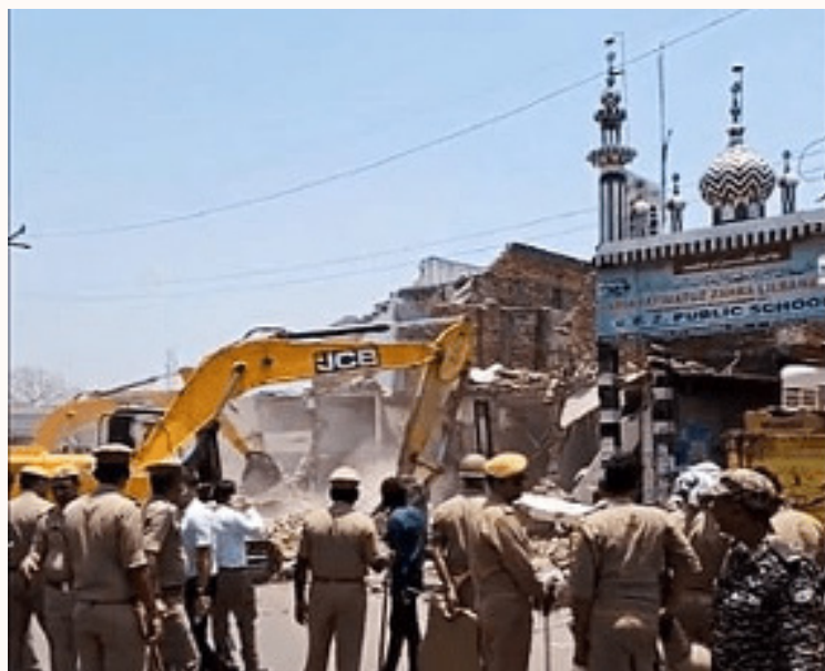
A demolition drive in Uttar Pradesh’s Akbar Nagar
