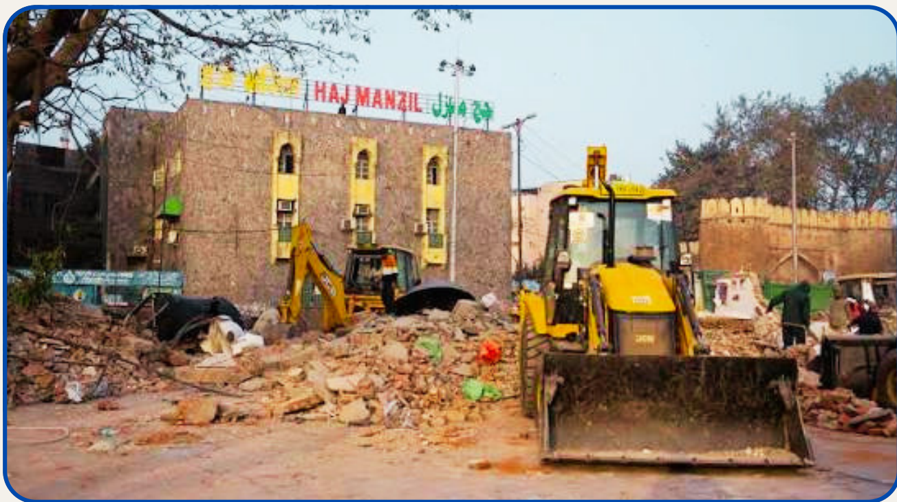
Demolitions near century-old mosque at Turkman Gate | Photo: Muhammed Shahamath/ Maktoob
